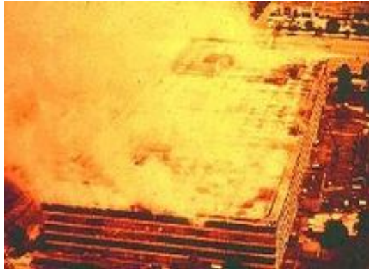
This aerial view of the 1973 fire gives you an idea of the intense conflagration that consumed the sixth floor of the NPRC building in St. Louis. (Photo courtesy Wikipedia.)
